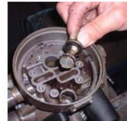
Carbon build up in an air dryer
